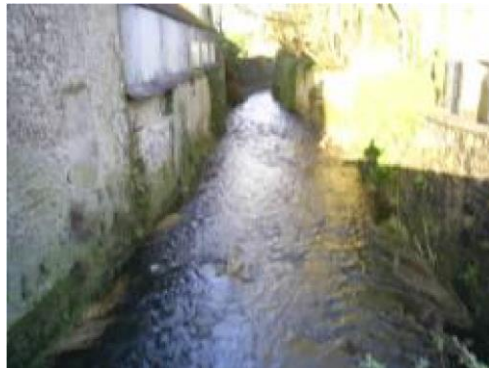
12. Reach 3: Final section of reach before confluence of Bregagh with River Nore. Note canalised channel and shading.
